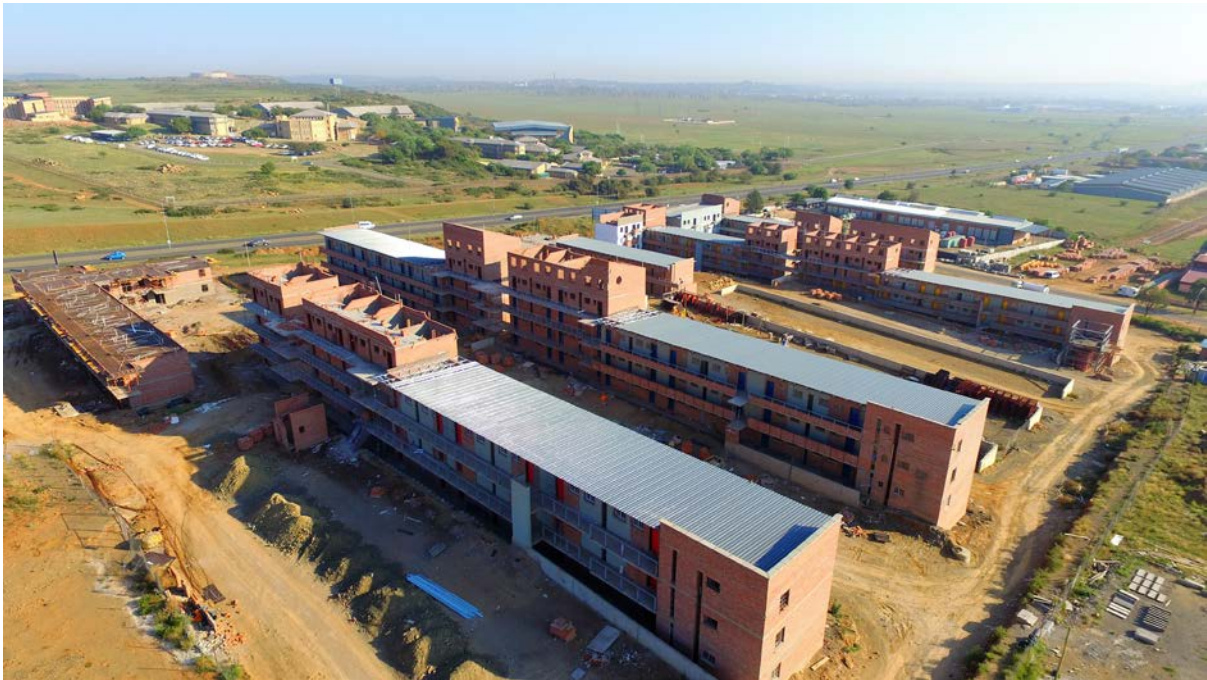
Figure 10: Hillside View Social Housing Progress
