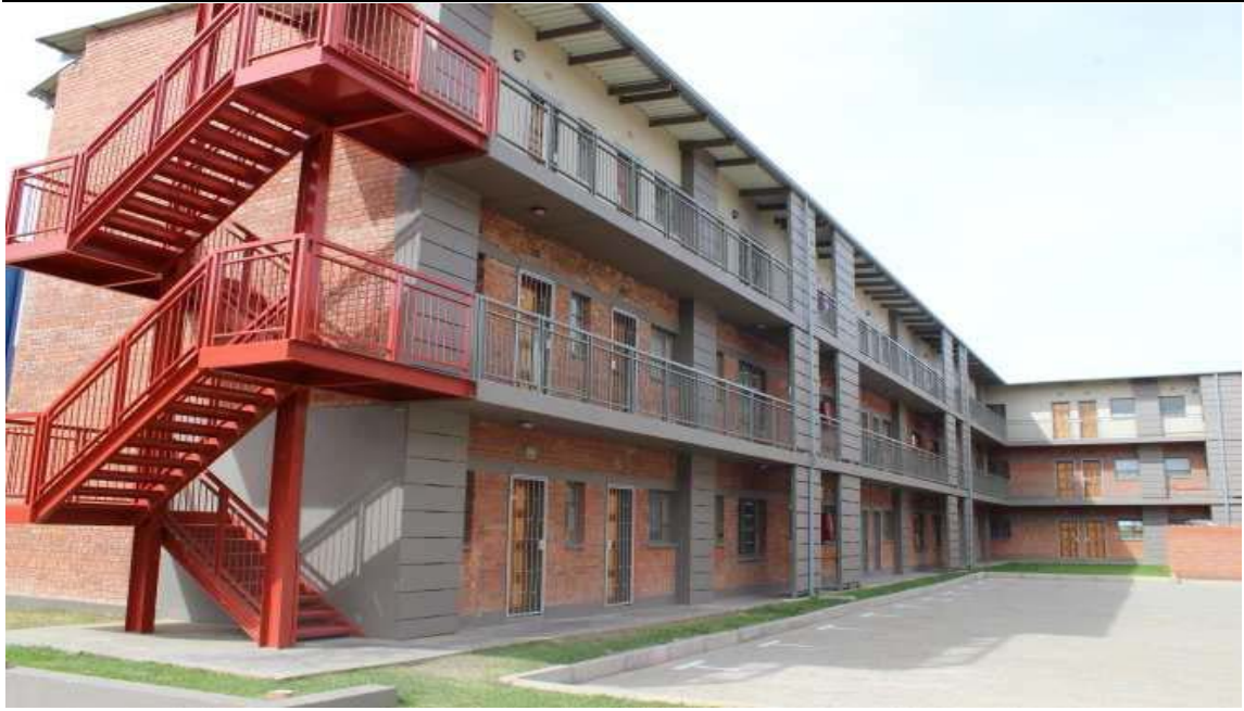
Figure 9 : Completed Units of the Brandwag Social Housing Project
